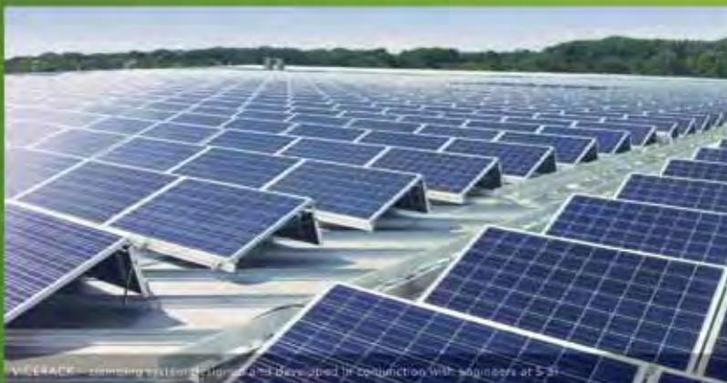
VICERAIL – connecting brackets securely corrugated metal roof deck with proper weather seal, etc.
